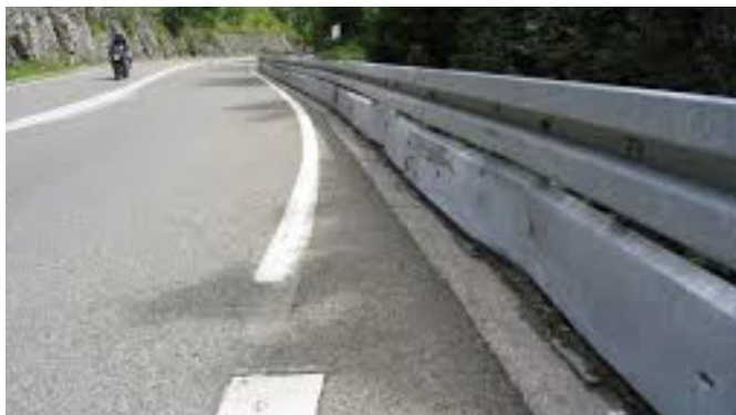
Figure 4.56 Modified U-shaped posts and attached to a curved concrete barrier
