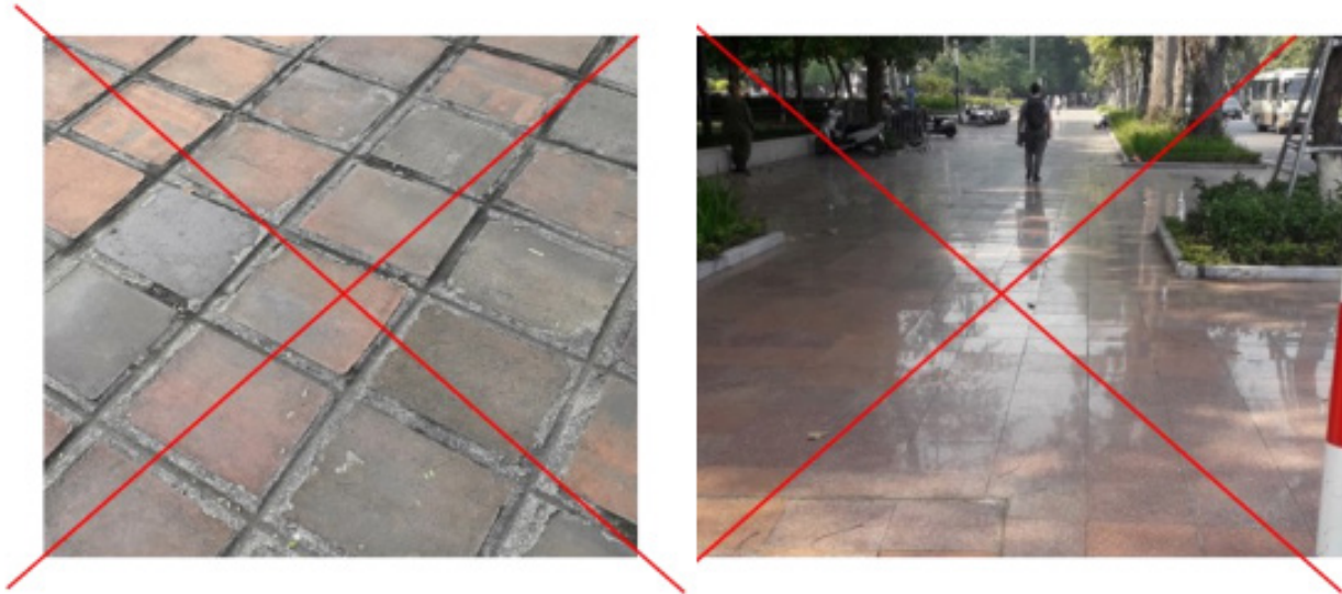
Figure 4.2: No tripping hazards or slipper floors.
