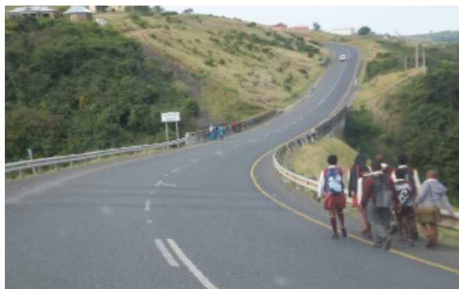
Figure 4.11: Unprotected footpath on rural national road.
