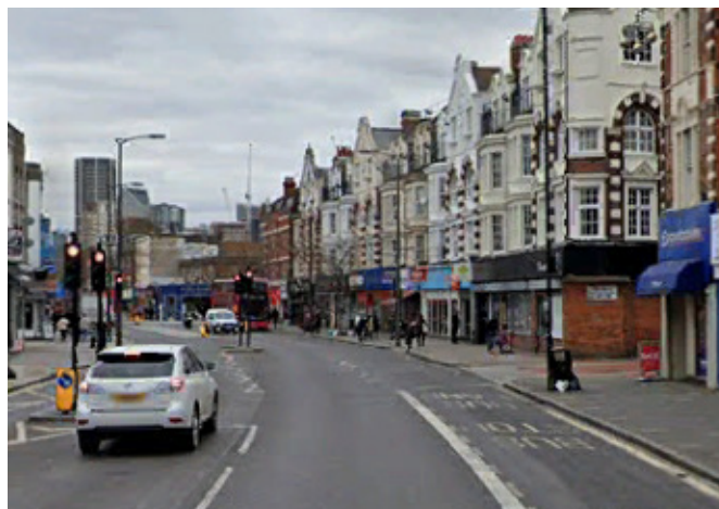
Figure 4.64: Bus lane and priority signal—UK.
