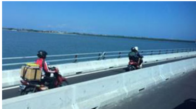
Figure 4.55: Concrete barrier-separated motorcycle lane in Indonesia.
