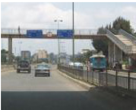
Figure 4.15: Grade separated footbridge—Ethiopia.
