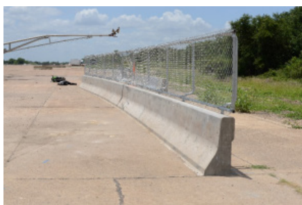
Figure 4.56 Modified U-shaped posts and attached to a curved concrete barrier
