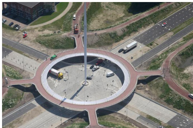
Figure 4.45: Floating roundabout for cyclists—Netherlands.
