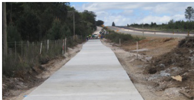
Figure 4.12: Segregated pedestrian/nonmotorized transport facility on rural road.
