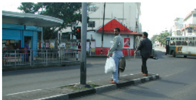
Figure 4.25: Lack of pedestrian space on median—mauritius—safety inspection.
