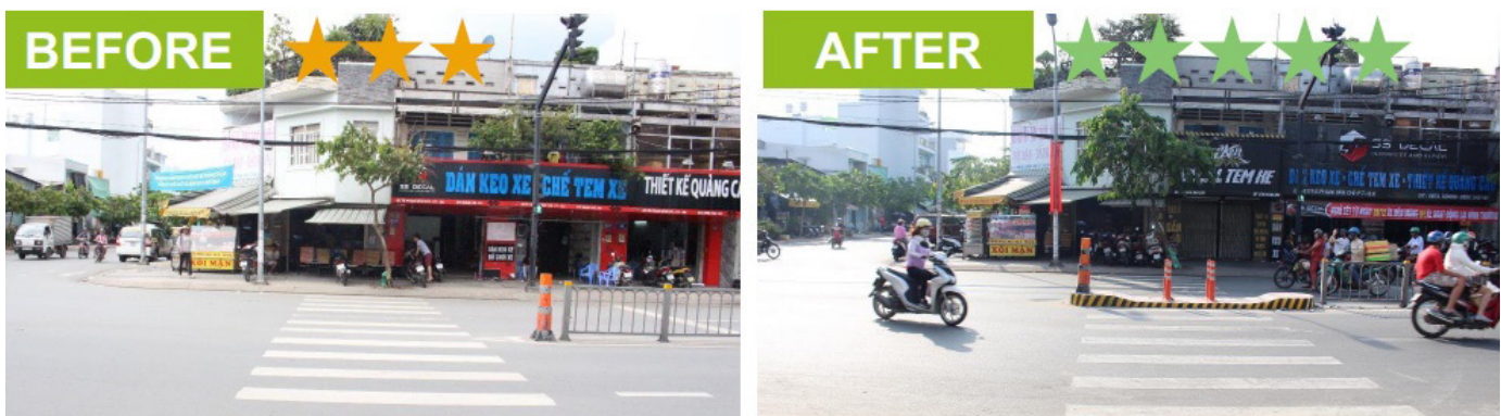
Figure 4.28: Installing pedestrian refuge—Vietnam.
