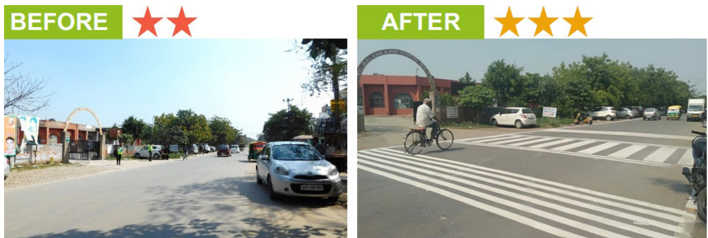
Figure 4.47: Installing crossings with advance cycle stopline—India.
