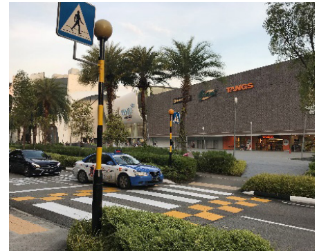
Figure 4.22: Well defined crossing with signing—Singapore.
