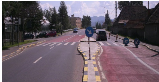
Figure 4.26: Painted and narrowing approach to crossing.
