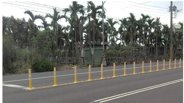
Figure 3. Flexible plastic delineator posts provide visual and tactile separation of traffic streams (Taiwan). Photo: Z7504/Wikimedia Commons
