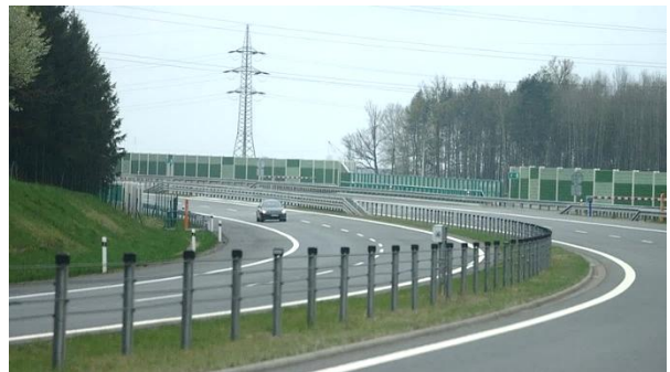
Figure 5. Cable median barrier (Czech Republic). Photo: Aktron/Wikimedia Commons
