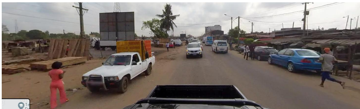
Figure 1. The absence of sidewalks puts pedestrians in conflict with motorized traffic., Highway P208, Abidjan, Côte d'Ivoire (Image: Google StreetView)
