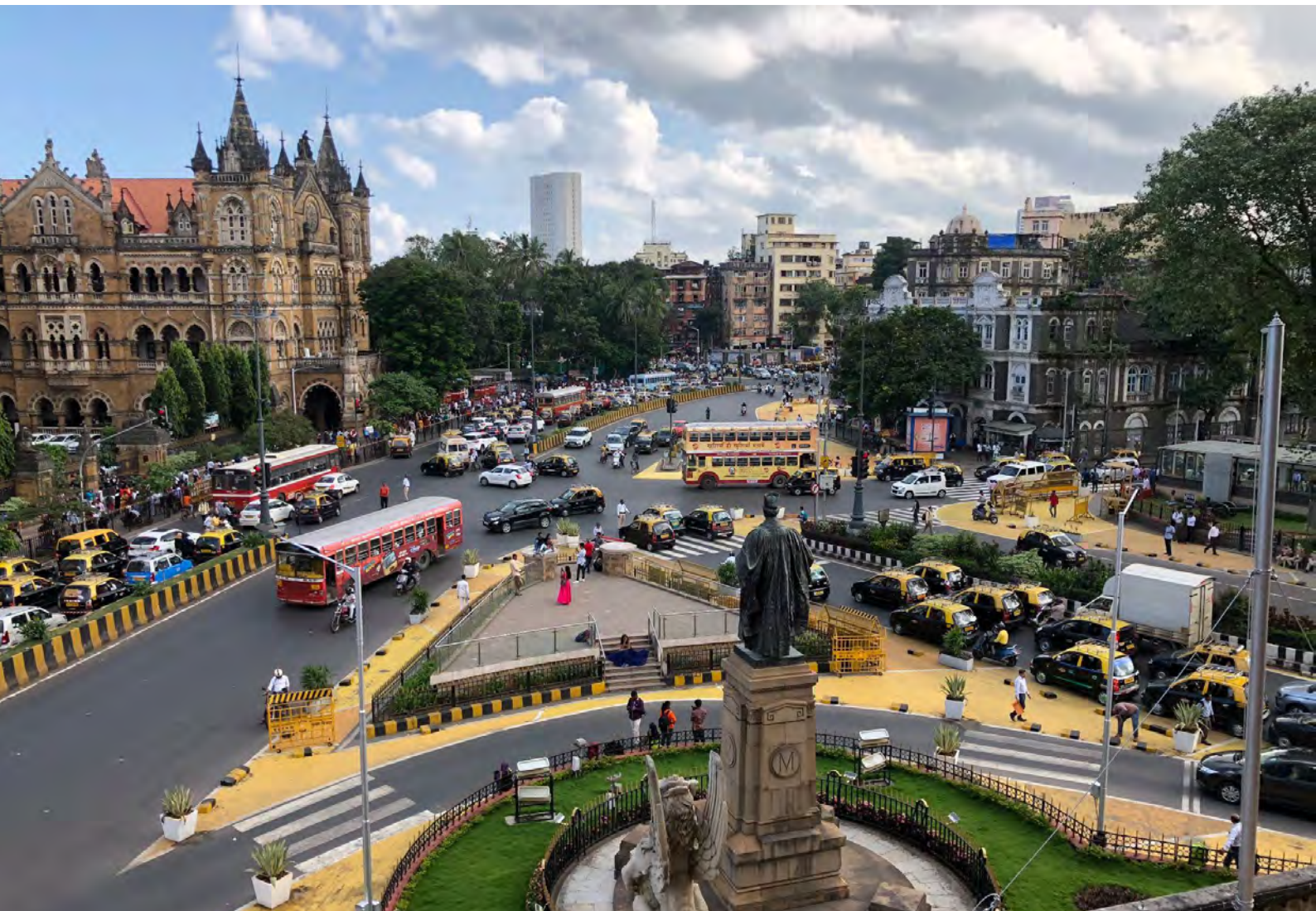
The photograph illustrates the intersection improvement efforts at Chatrapathi Shivaji Maharaj Terminal (CSMT) in Mumbai. This project utilizes interim/tactical urbanism strategies to enhance Road safety and accessibility for all the users at the intersection. Photo credits : GDCI
